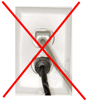
Two cords plugged into the same circuit is not recommended.
